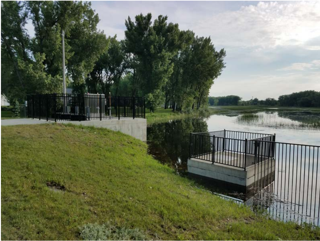
East side of Tavis Road, inflow to reduce levels
